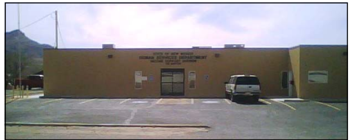
The newly-renovated T or C ISD Office.
